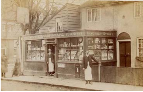
Lamorbey Post Office and Stores, Halfway House Sidcup
