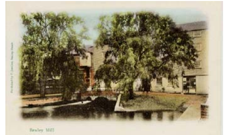
Bexley Mill, High St Bexley
