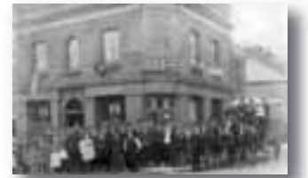
Rose and Crown, Bexley Road, Erith. Ceased trading in 1967 to make way for town centre redevelopment.
